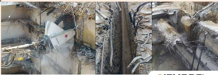
▲ A DMW 220 cutter wheel being used to cut through a 900 mm thick concrete floor containing 30 mm diameter rebar laid in a tight pattern.
