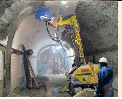
A DMW130 mounted on a Liebherr tunnelling excavator profiling a tunnel at predetermined intervals for the installation of water drainage piping and support arches.
