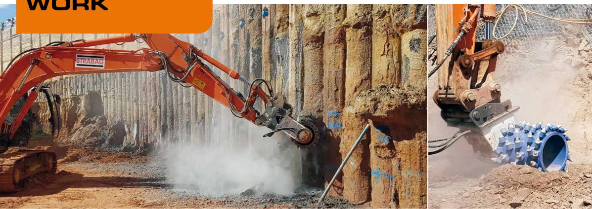
▲ The surface layer of concrete drill piled wall are profiled to a high degree of accuracy using an ES 60 HD fitted with a cutter drum.
