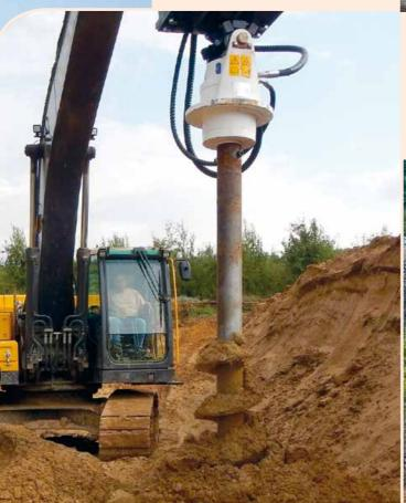
An EBA 2300-D drilling 5 m deep holes for the in tion of a retaining wall.
