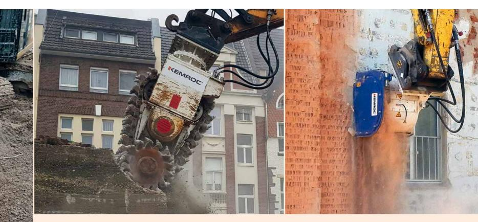
Demolition of a bunker using an EK140 chain cutter. The bunker is attached to another building and a low vibration method must be used to demolish it.
