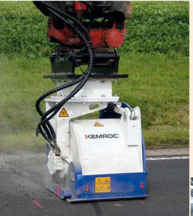
An **EX45HD** planing a 4 cm deep strip from an asphalt surface. The rotation module allows the planer to work in a direction at an angle to the axis of the excavator.
