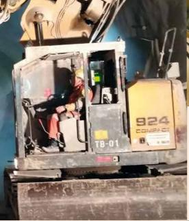
▲ An **EX45HD** planer with tiltrotator removing a 12 cm deep layer from the brick lining in a tunnel. A plastic damp proof layer will be applied to the accurately profiled surface afterwards.
